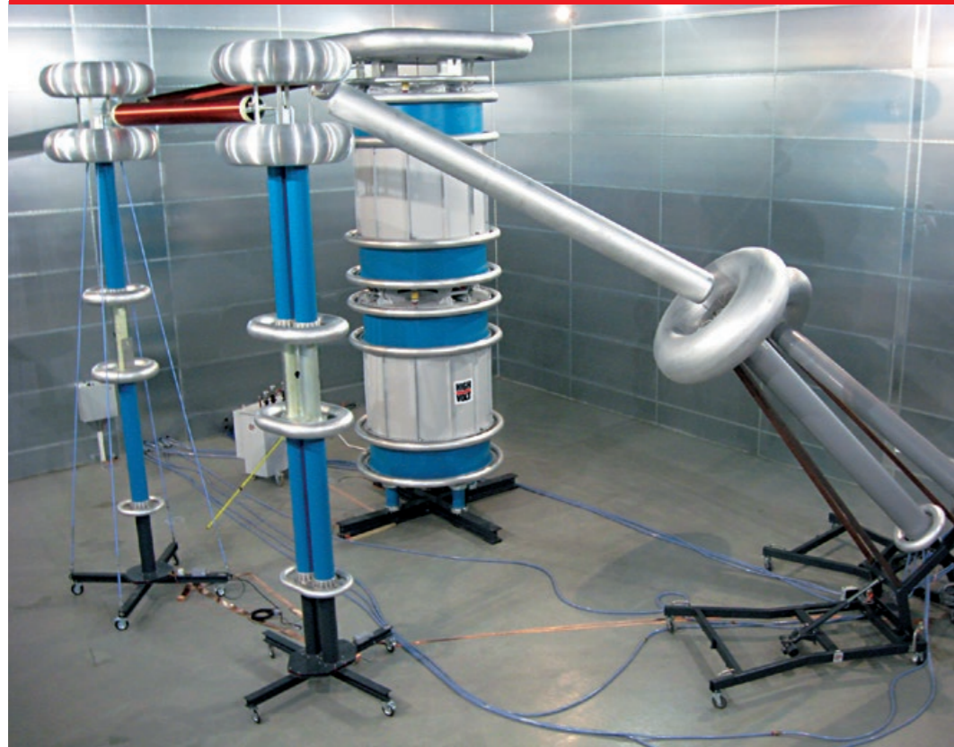
Fig. 1 Test field for 500 kV cables with routine WRM test system with 800 kV and 28,000 kVA
