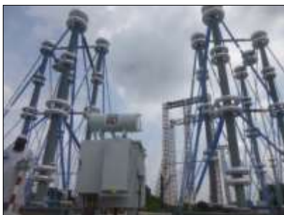
Fig. 2: Outdoor HVDC test system type FGP 200/1200 (200 mA, 1200 kV); Manufactured by HIGHVOLT
